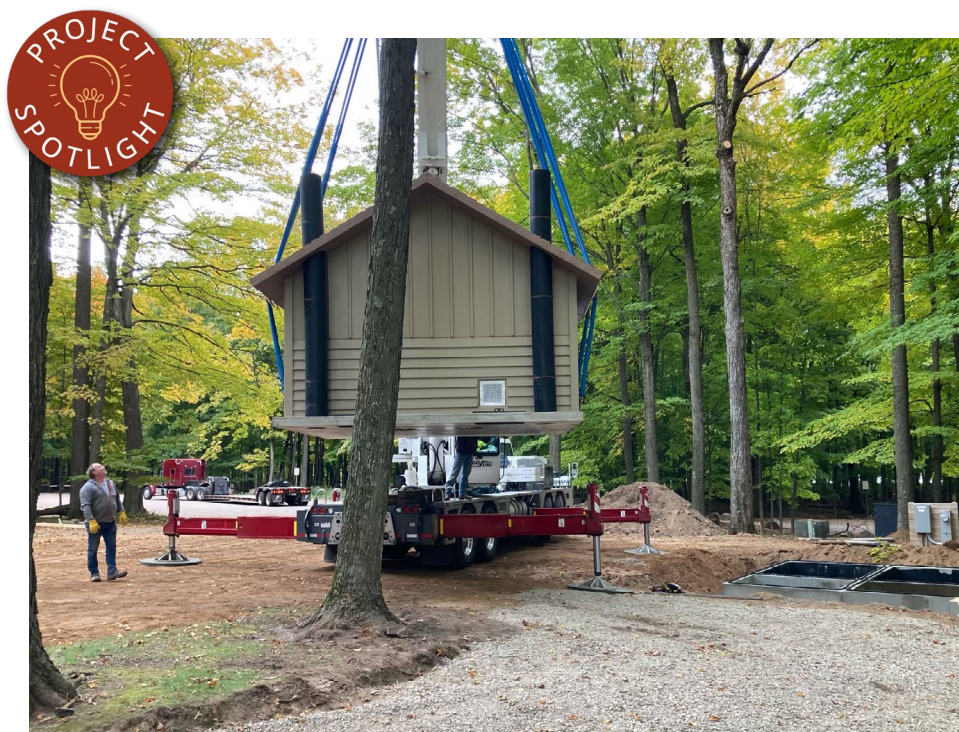
Installation of the new privy at Cherokee County Park.
