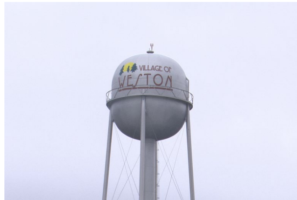
Water tower in Weston
