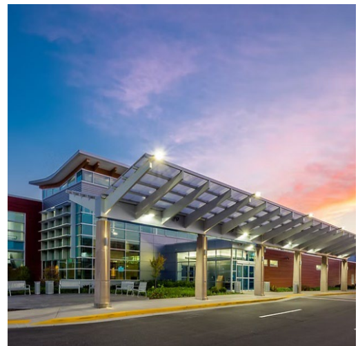
Central Wisconsin Airport
