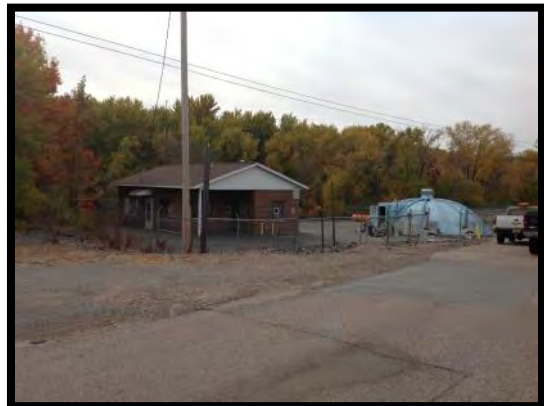
Brokaw Wastewater Treatment Plant
